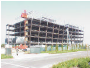
EFI Building B September 2000
