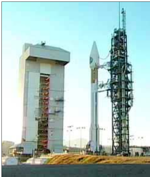
File image of SLC 3-E shows the mobile service tower (left) and umbilical tower (right). Photo: NASA TV/Spaceflight Now
