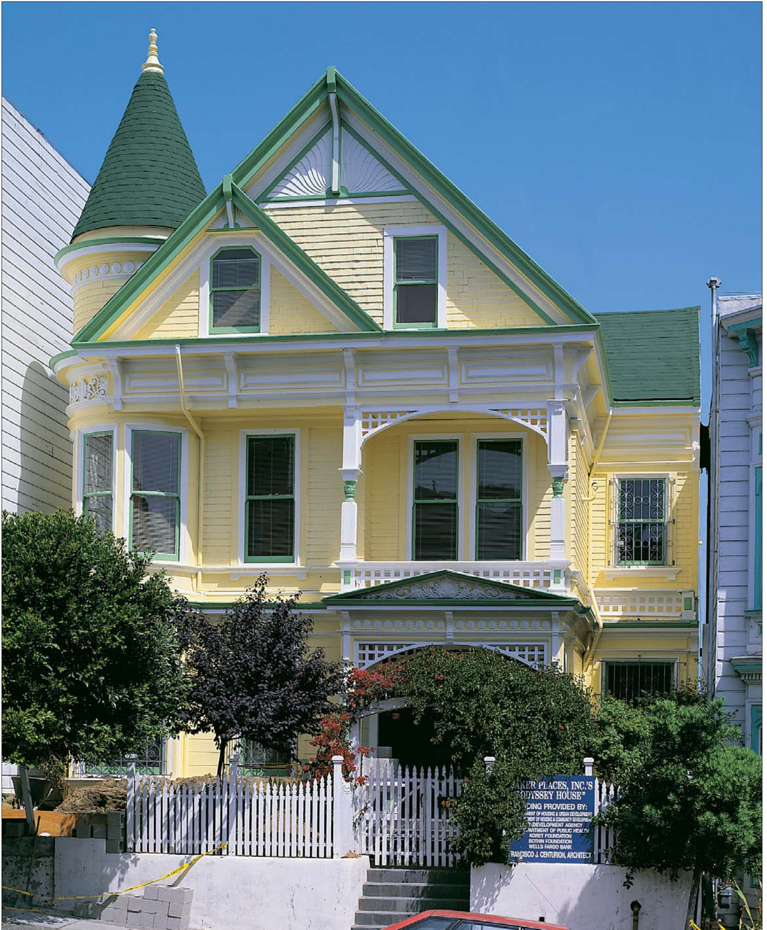
This cheerful yellow house on Oak Street near Laguna is a classic Queen Anne, with a round turret, asymmetrical façade, and a sunburst in the gable, but it has one unusual feature: a second-story veranda, matching the design of the porch below it.
