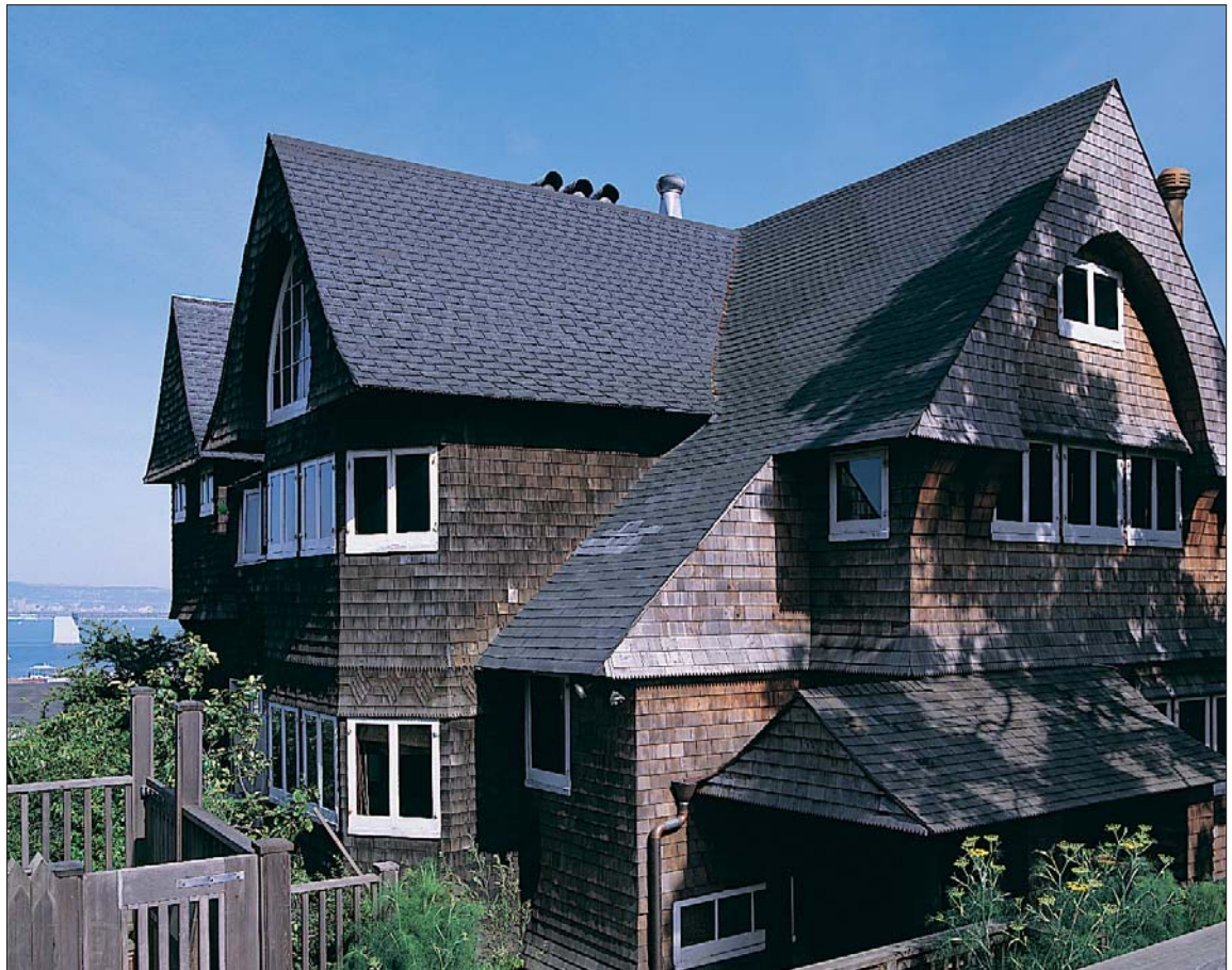
The Horace Livermore house (top) was remodeled by Willis Polk, who then built his own house (above) just behind it. Two of the four Worcester cottages (center left) complete an exclusive enclave on Vallejo Street at the top of Russian Hill, one of the most historic sites in the city.
